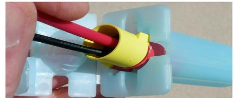
**Step 6** – Close the lid of the tube to apply pressure onto the insulation of the wires. This ensures that the wires will not slide out when they are pulled-upon during system maintenance. Place small diameter wires in the same channel as the larger wires so they are captured securely by the tube lid.
