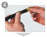
Immediately insert the expanded pipe end into the fitting until it reaches the last and largest ridge. Note the pipe contracts over time due to the PEX memory effect.
