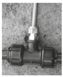
**5. Fully installed**The fitting is now fully installed.
