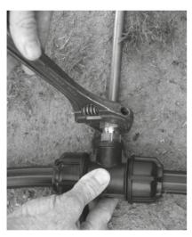
**4. Nut tightening**The nut should be tightened firmly with a wrench.
