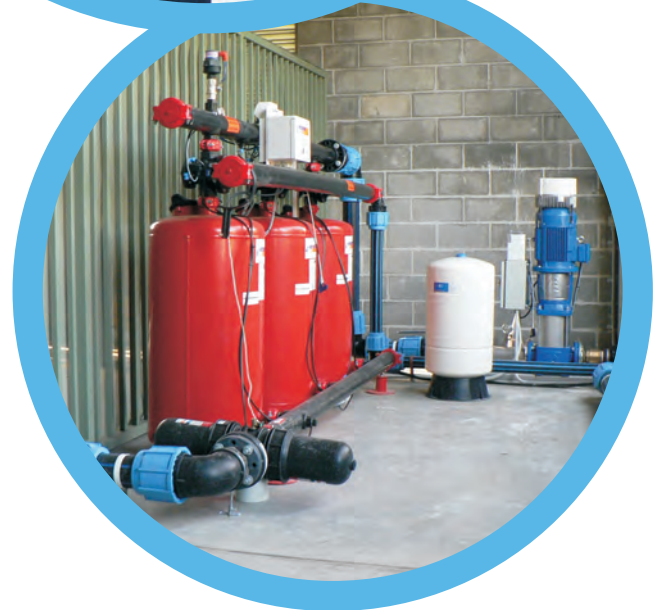
The gravel filter automatically back flushes which helps improve system efficiency
